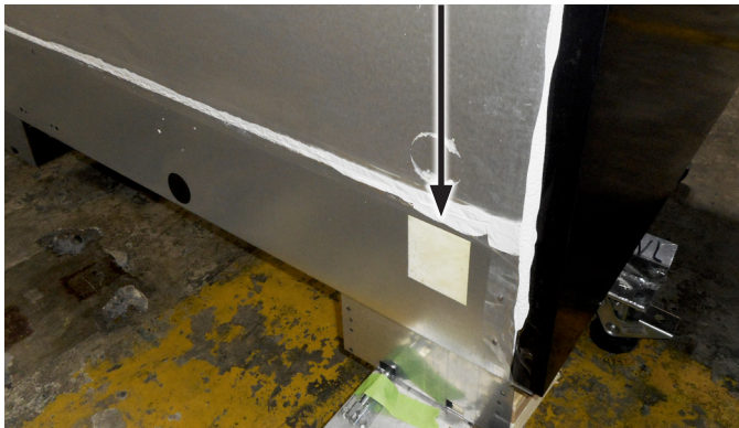
FIGURE 38: Rear Wall Opening for Water Lines (Exterior)
