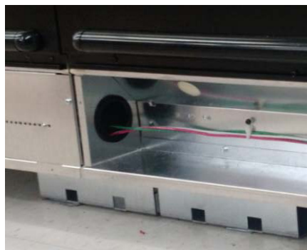
FIGURE 51: Case-to-Case Wiring
