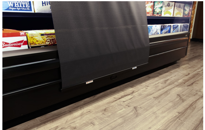
FIGURE 32: Night Curtain Pulled Down
