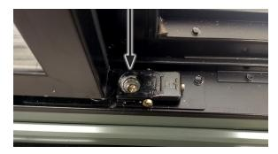
FIGURE 33: Torque Adjuster Plug
