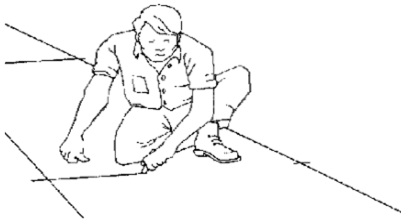
FIGURE 5: Measure and Mark Exact Case Outline
