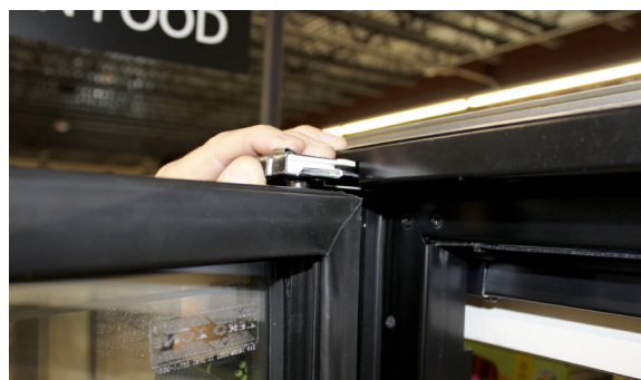
FIGURE 27: Push Door & Hinge Pin into Place
