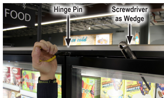
FIGURE 26: Use a Wedge & Pinch Hinge Pin
