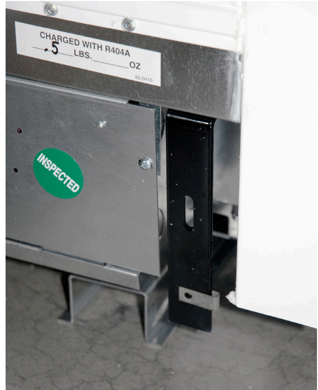
Install Tinnerman clip to each bumper support (over the round hole).
