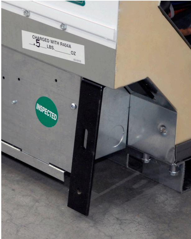
Install Tinnerman clip to each bumper support (over the round hole).
