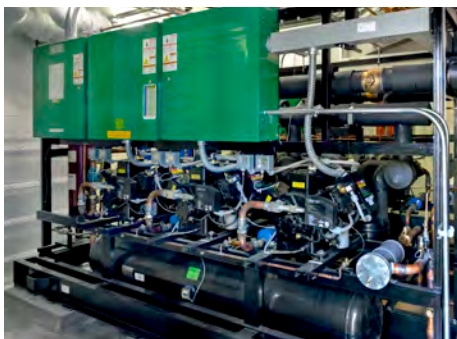
Synthetic Refrigerant Chiller
